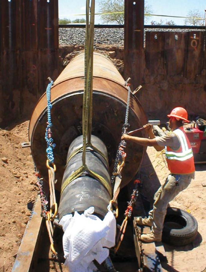
The three contractors are installing large diameter steel casing.
